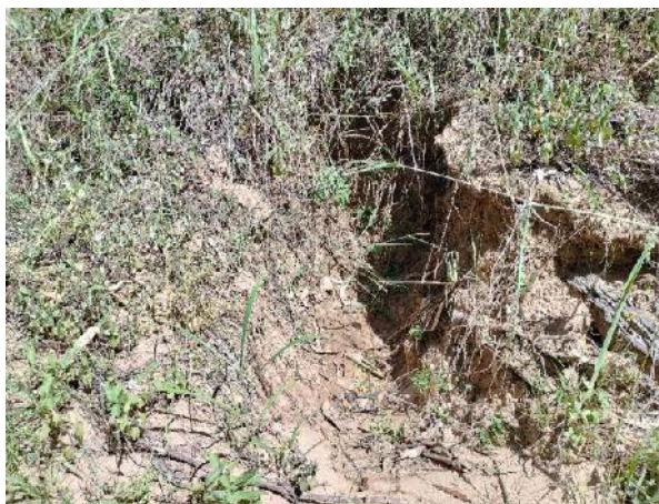
Figure 12: Large crack in bank
