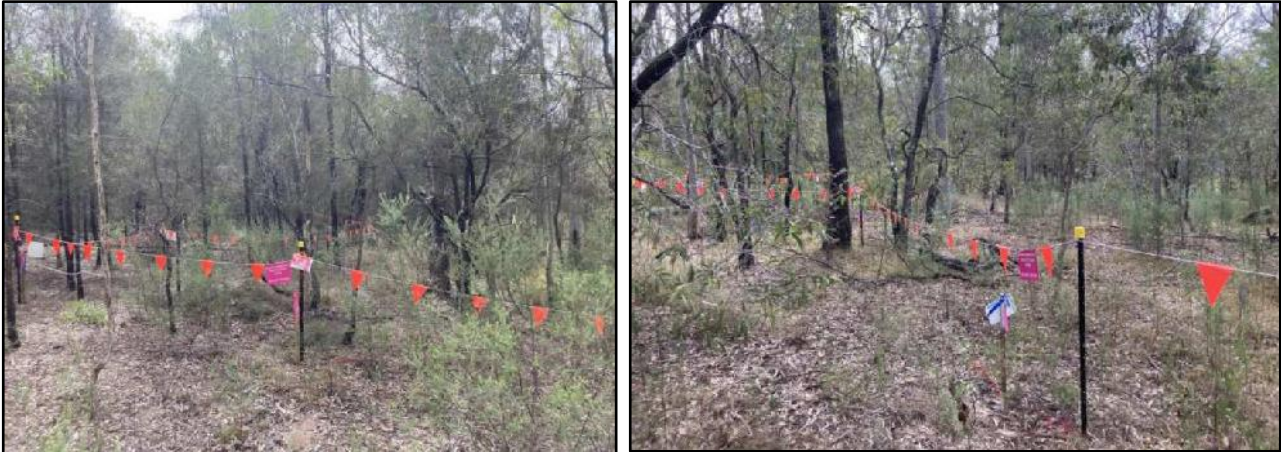
Photo set 1: Temporary fauna friendly tree protection fencing.
